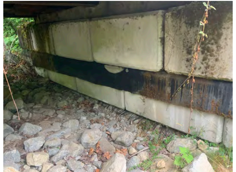
Left Bank Abutment when facing downstream
