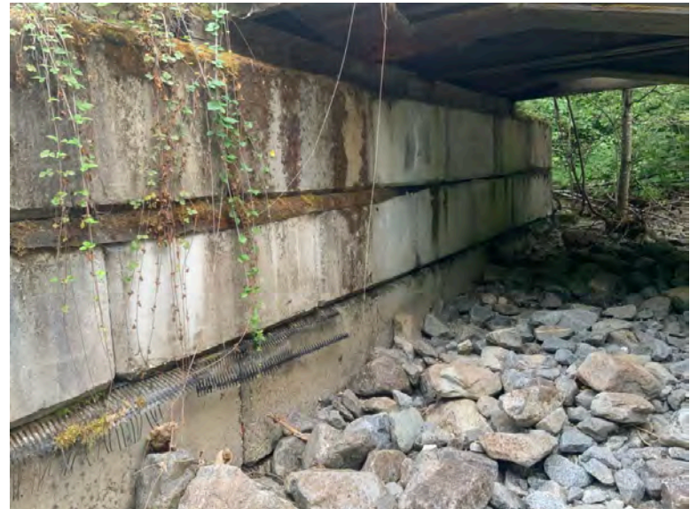
Right Bank Abutment when facing downstream
