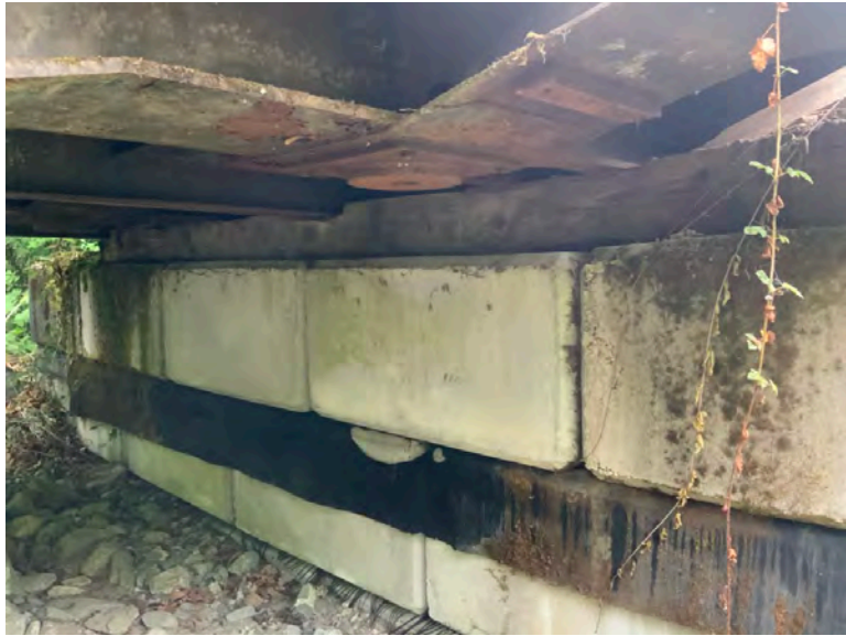
Left Bank Abutment when facing downstream
