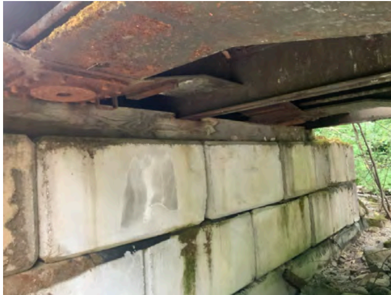
Right Bank Abutment when facing downstream
